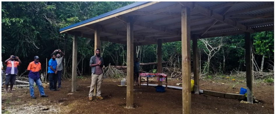
Building a ferrous cement tank connected with guttering to an existing community hall in Hog Harbour, Vanuatu as part of the Department of Water Resources Plumbers Training
