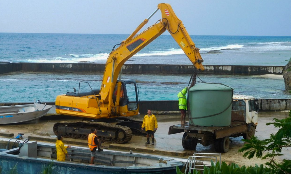
Water tank delivery by boat to Mauke. Photo: Bruce Corbett.
