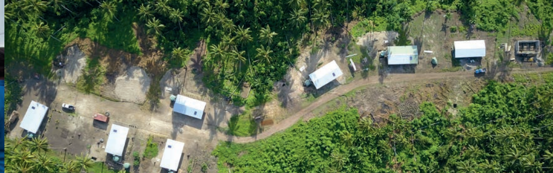
A drone view of the development. Photo: Gordon Botha
